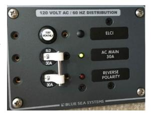
SHORE POWER supports all AC equipment and receptacles on board, as well as the inverter/battery charger.
