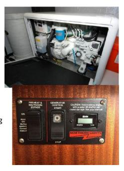
Let the generator warm up for about two minutes, and then at the AC control panel, move the sliding protector up and energize the generator power breaker. Then turn on AC systems as you would on shore power one system at a time. Monitor your current usage amp draw.
