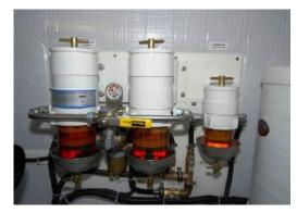
Check the two fuel filters for contaminants or water as part of the pre-cruising engine room check. If there are contaminants or a separation of fluid in the bottom of the glass collection containers, they should be drained of the contaminants as follows:
