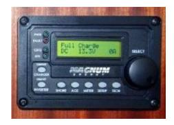
the units' Inverter converts DC battery power to AC power to supply all AC outlets on board with 110V AC. Note: The inverter does not provide AC power to the water heater or the electrical heating units.
