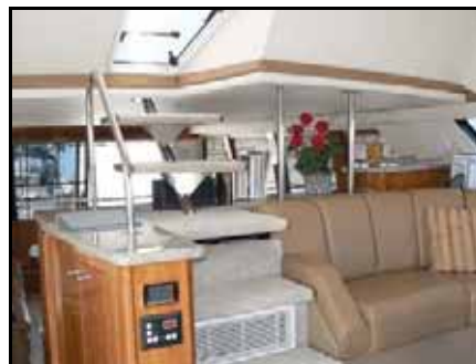
Steps to the flybridge with the AC power panel cabinet at their base...
