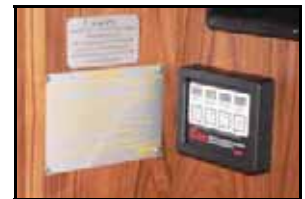
(Above) The Force 10 Range (Below) The Propane monitor & solenoid control panel.
