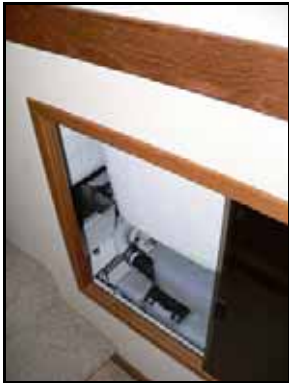
One of the two equipment access cabinets in the companionway.
