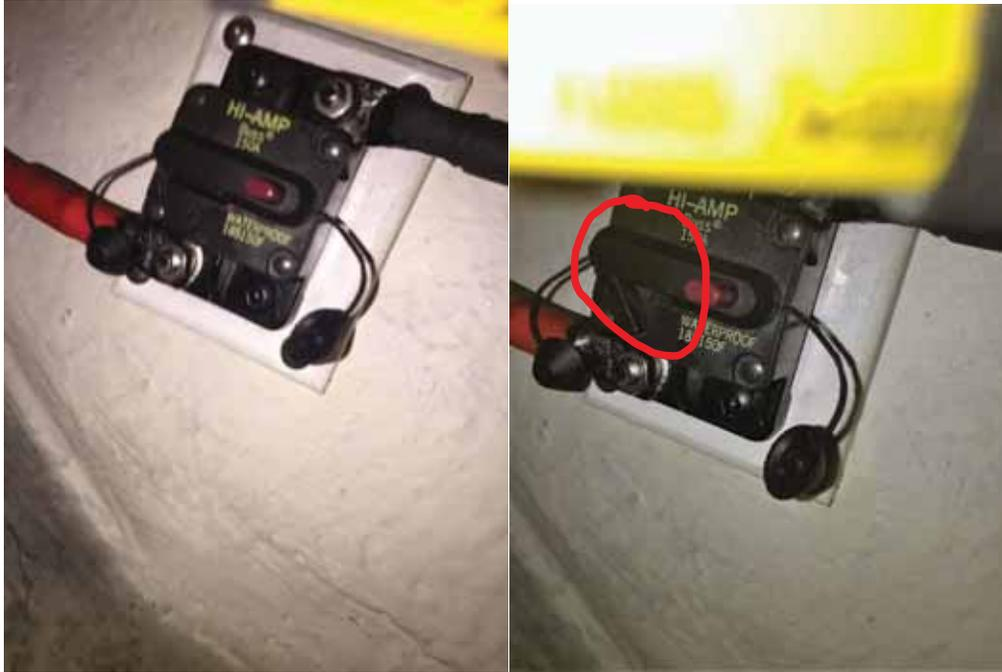
the Bow Battery. Here are two photos of the Bow Thruster breaker. The left photo shows the breaker in the normal, “closed”, position and the right photo shows the breaker “open” with the breaker lever circled in red. If the Bow Thruster stops working, check this breaker and close the lever if necessary. The red button is the TEST button it is NOT the breaker lever. The breaker lever is black and to the left of the TEST button—again, circled in the picture above at right.
