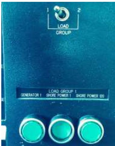
Switches set for shore power 1 and transfer switch on which routes power to load group 1 and 2. Meter set to group 1.
