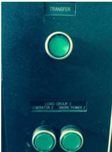
The transfer switch provides power to both load groups. Regardless of source.
