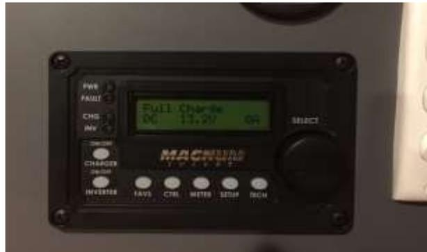
***Inverter:*** When at anchor or not plugged into shore power, AC power is made available only when the inverter breaker is on and the *inverter* button on the Magnum battery controller (located above the electrical panel) is on. The inverter breaker(#22) is located on the AC 120 volt electric panel and should always be left on.
