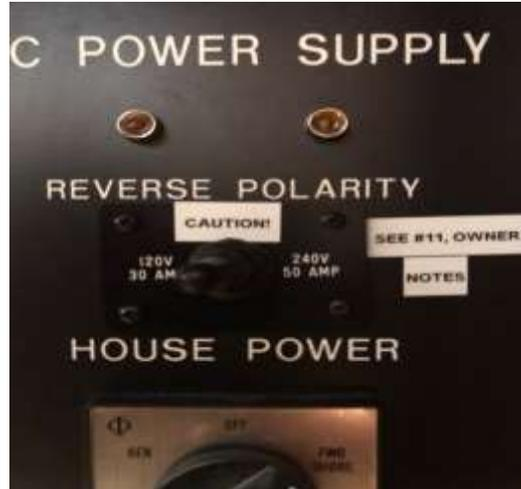
**THIS TOGGLE SWITCH MUST BE SET TO THE PROPER VOLTAGE YOU ARE CONNECTING TO AT THE DOCK, EITHER 120V OR 230V, (BEFORE YOU FLIP ON POWER WITH THE BREKER). FAILER TO SET THE TOGGLE SWITCH FROM 230V TO 120V WHEN PLUGGING INTO A 120V 30A POWER SOURCE WILL FRY THE 30A RELAY.**
