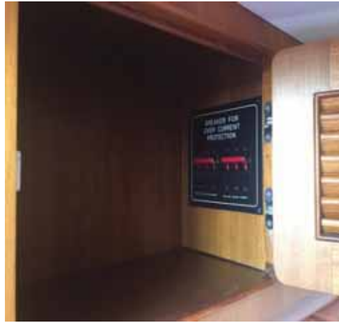
Forward: Master Berth Main House breaker
