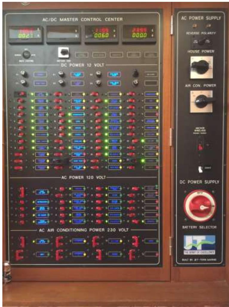
When not connected to shore power or running the generator, the AC power and outlets will only function if the *inverter* button on the Magnum battery controller is on (see: 5. Batteries Charger/Inverter). The battery charging breaker(#17) located on the AC Power 120 Volt electric panel should always be left on.
