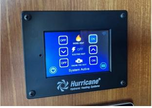
use the electric heat elements, you use the arrows to toggle between OFF, 1.5kV, and 3kV. The appropriate AC breakers also must be on, and shore power is required for electric heating.
