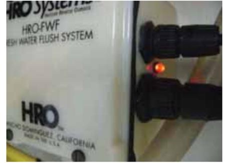
14. Once the fresh water flush LED goes out, flip off Watermaker circuit switch in engine room and shut down the genset if not needed for other reasons. Close the thru hull valve. Open the high pressure valve to its fully counterclockwise position.
