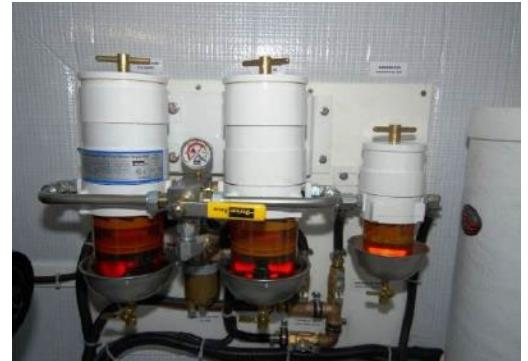
Check the two fuel filters for contaminants or water as part of the pre-cruising engine room check. If there are contaminants or a separation of fluid in the bottom of the glass collection containers, they should be drained of the contaminants as follows:
