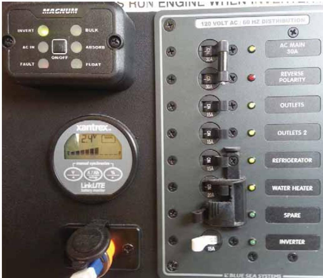
The box at the upper left is the inverter used to send 120V power through the system. Do NOT turn it on unless on shore power or the engine is running. The 1200 watt inverter that can power ac loads from the batteries. High load devices (microwave, coffee pot, special hair dryer) put a considerable drain on the house battery bank and the engine should be run during inverter use to relieve the load on the batteries.
