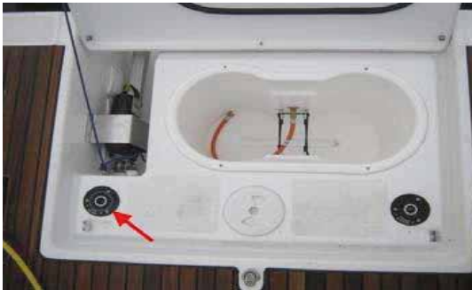
Aft Water Tank Fill Port (red arrow)
