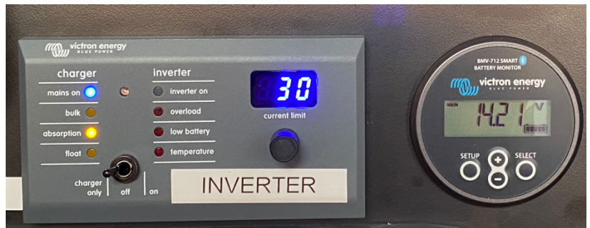
FIGURE 2 - SWITCH LEFT (NORMAL) / RIGHT (INVERTER)
