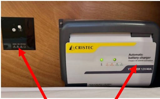
GFI Breaker and Battery Charger
