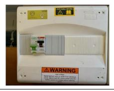
Aft cabinet AC Ground Fault Breaker
