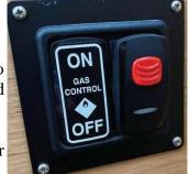
lighting the stove or broiler it takes about 3-5 seconds to allow the thermocouple to sense the flame.
