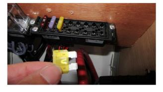
A fuse protects an electrical circuit from excess current. If it blows, you must replace it with another fuse of the same rating.
