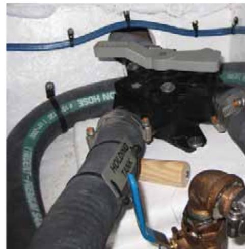
*A view of the Y-valve controlling movement of waste from the toilet with flow directed to the holding tank*
