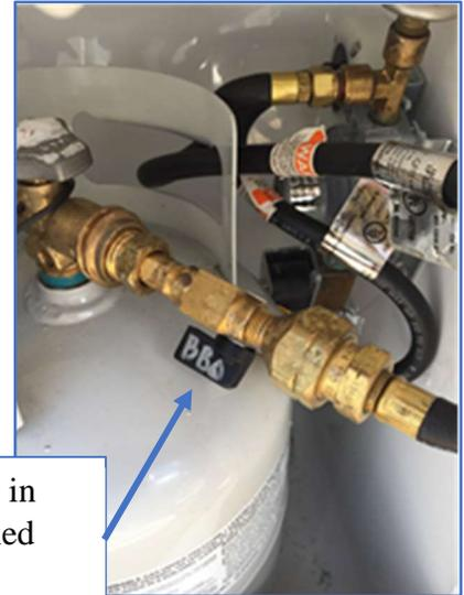
BBQ isolation valve in Open Position, aligned with pipe.
