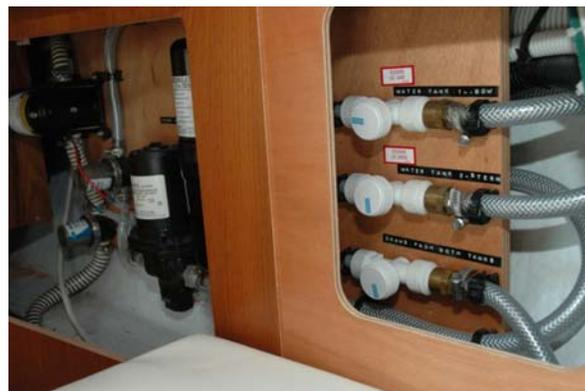
To best manage your water, we recommend drawing down one tank at a time. You can do this by running out of one water tank at a time. The picture above shows the **top valve rotated with horizontal lines pulling water from Tank 1. The other two valves are turned off in the “vertical” position.** Once you run out of Tank 1, you can switch over to
