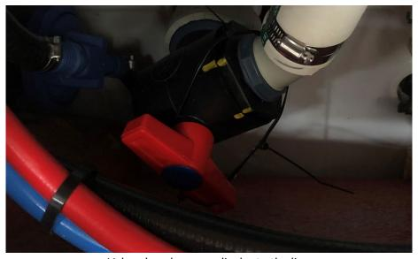
Valve closed, perpendicular to the line
