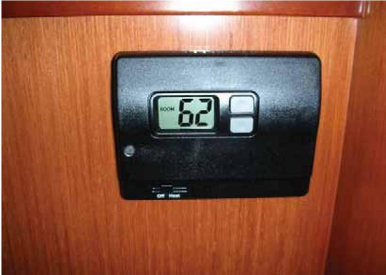
The heater outlets in all the rooms are controlled by baffles on the opening to regulate heat, except the salon which is regulated by the temperature set on the control unit.
