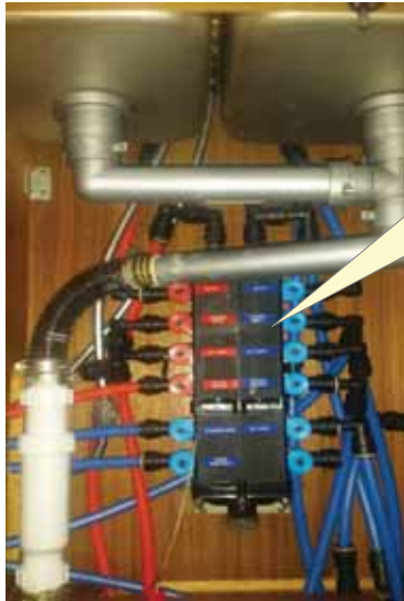
DOMESTIC WATER DISTRIBUTION SECTION SHUT OFFS
